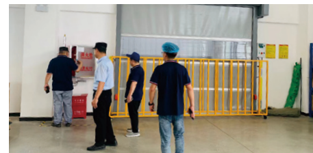
Work Safety Inspection - Firefighting Equipment
