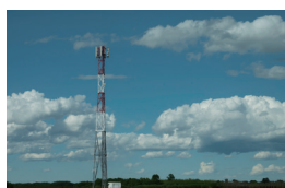
Telecom Base Stations
