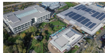
Commercial & Industrial Solution
