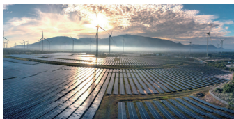
Source-Grid Side Solution
